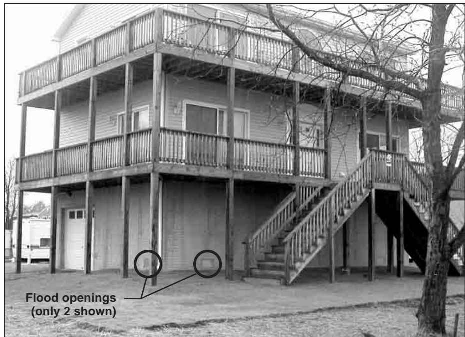
Figure 3. Full-height solid perimeter walls surrounding garage and storage area (only two openings visible)
