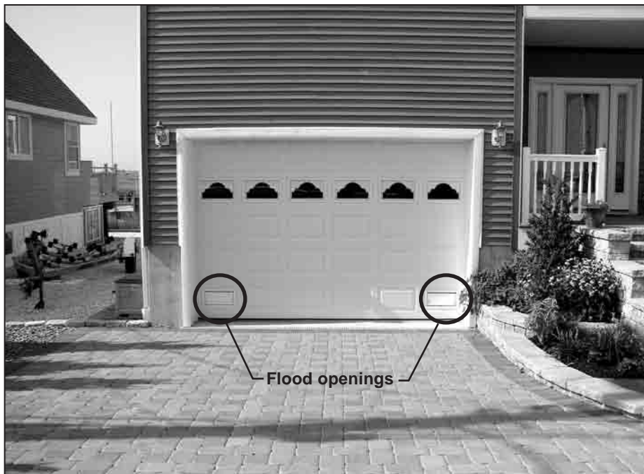
Figure 4. Attached garage, with engineered openings installed in the garage door
