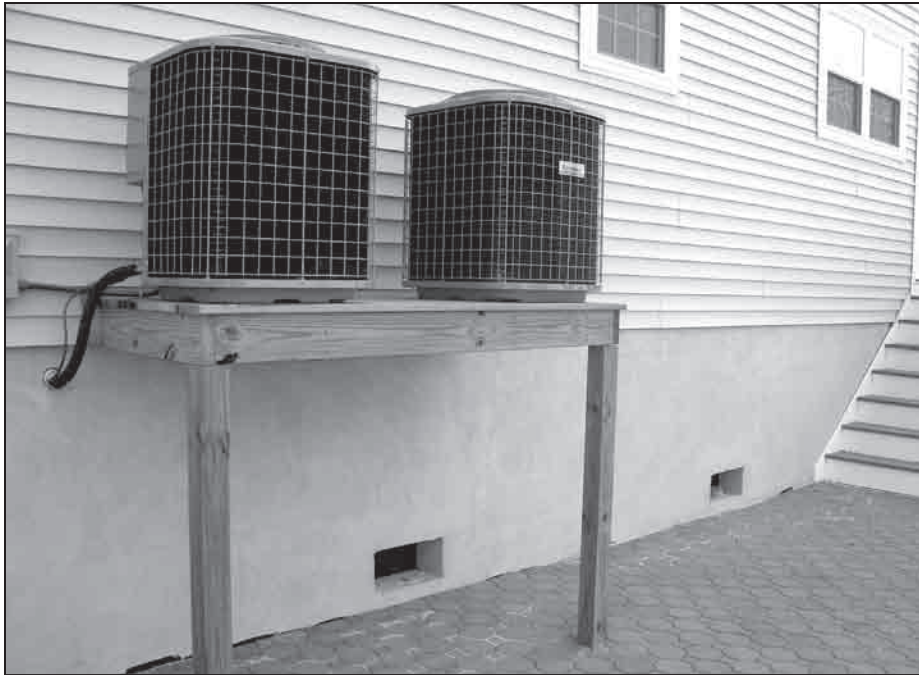
Figure 19. Foundation wall with omitted blocks as flood openings (insect screen not visible)
