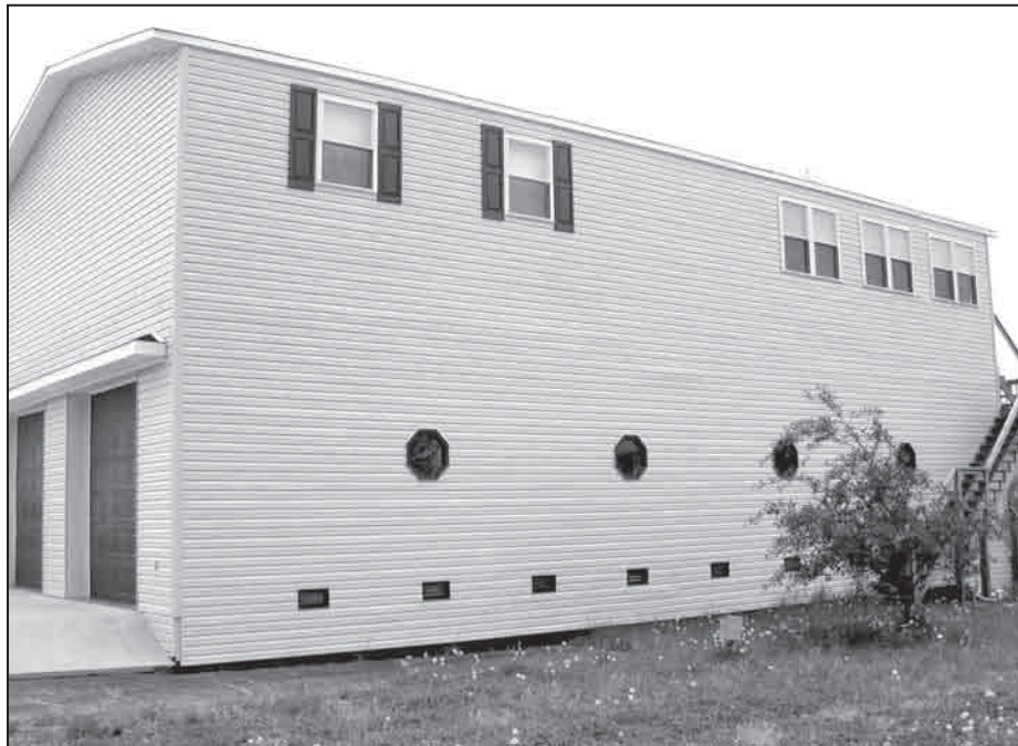
Figure 7. Manufactured home installed above a full-height framed garage (note elevation of driveway slab on left; the openings are within 1 foot of interior grade of the slab)
