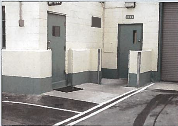
Figure 3-12. Front of retrofit dry floodproofed building where drop-in flood shields protect doors
