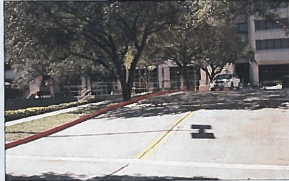
Figure 3-24. Ross Sterling Avenue was raised to protect the MSB to the level of the base flood (source: Walter P. Moore)
